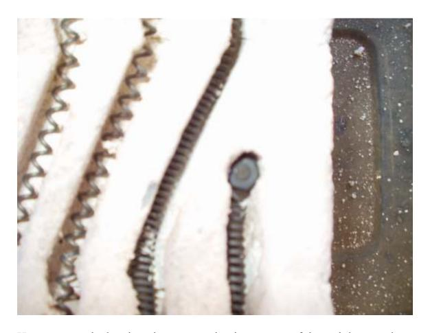
Here you see the heating element terminating on one of the stainless steel terminals before the paint is applied.
